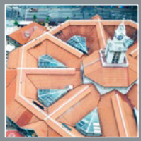
The cast-iron structure is also known as pasar besi (market of iron) in the Malay language.
